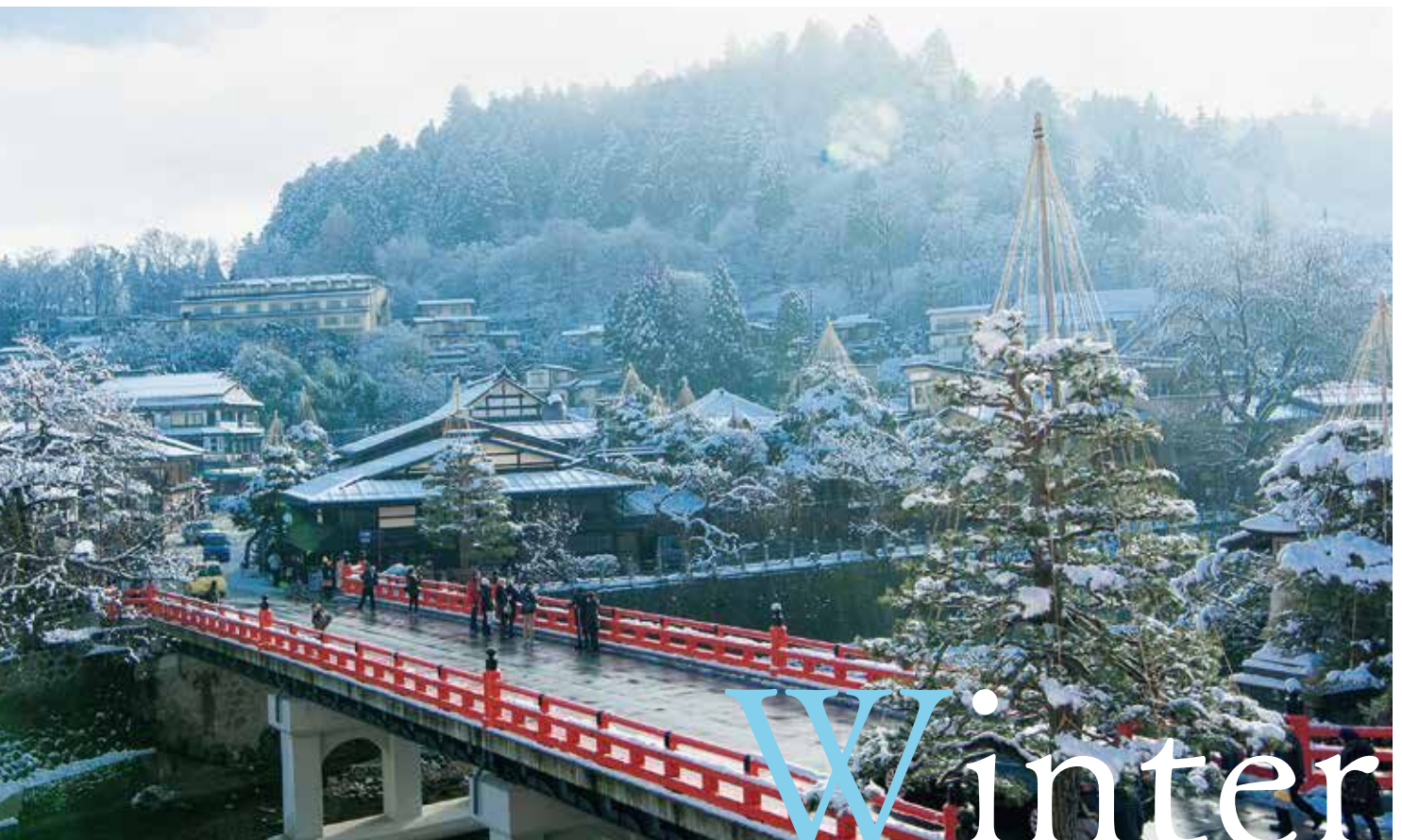
Nakabashi Bridge (Takayama)
